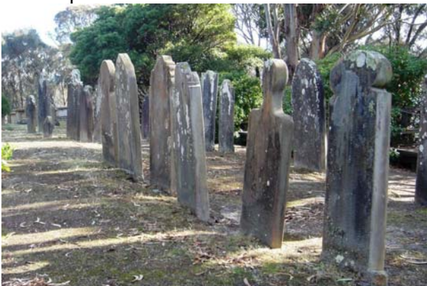
Most of the tombstones have deteriorated since the sandstone they were made of was not durable.
